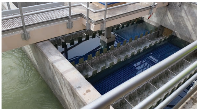
The high-rate sedimentation process tank allows ballasted flocs to settle up to 35 times faster than in conventional clarification processes.
