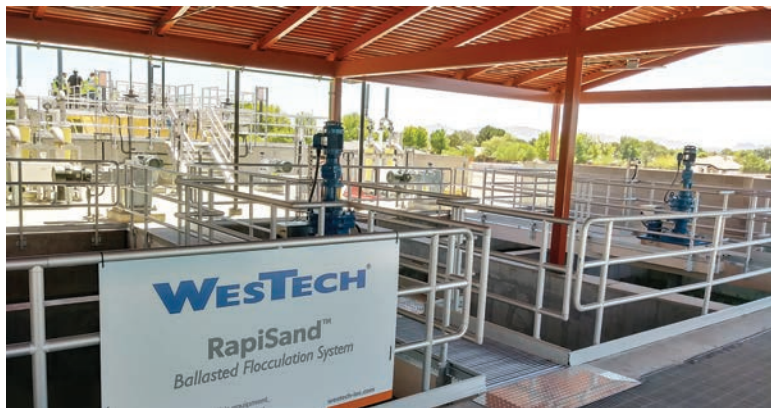
A double-train ballasted flocculation system doubled treatment capacity for a low cost.
