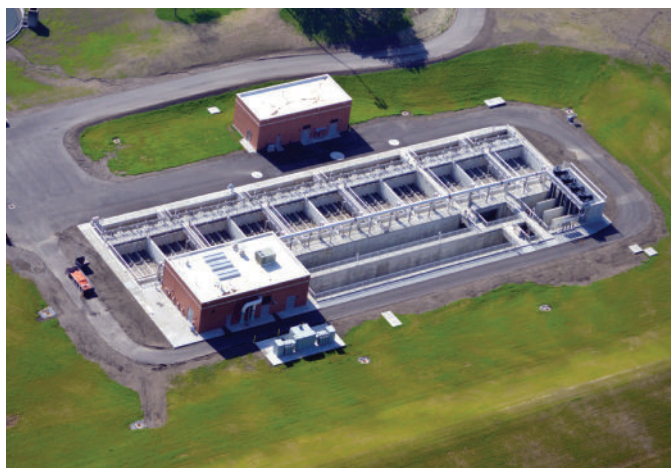
Aerial view of high-rate treatment facility
