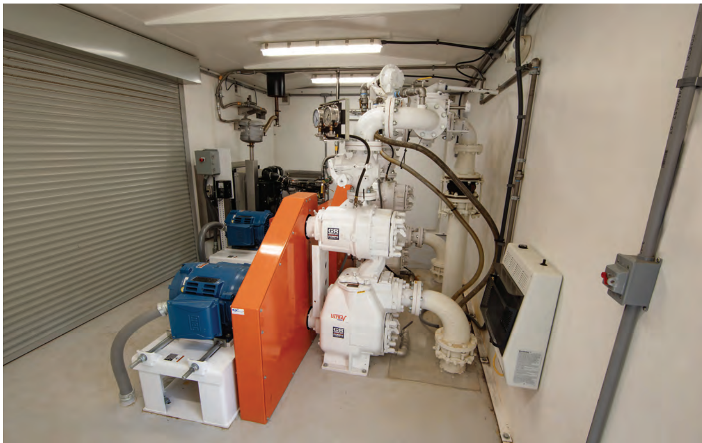
The enlarged size of modular enclosures provides added space for performing routine pump maintenance while shielding operators from external conditions. Oversized roll-up doors allow access to station components should heavier-duty lifting equipment be required.
