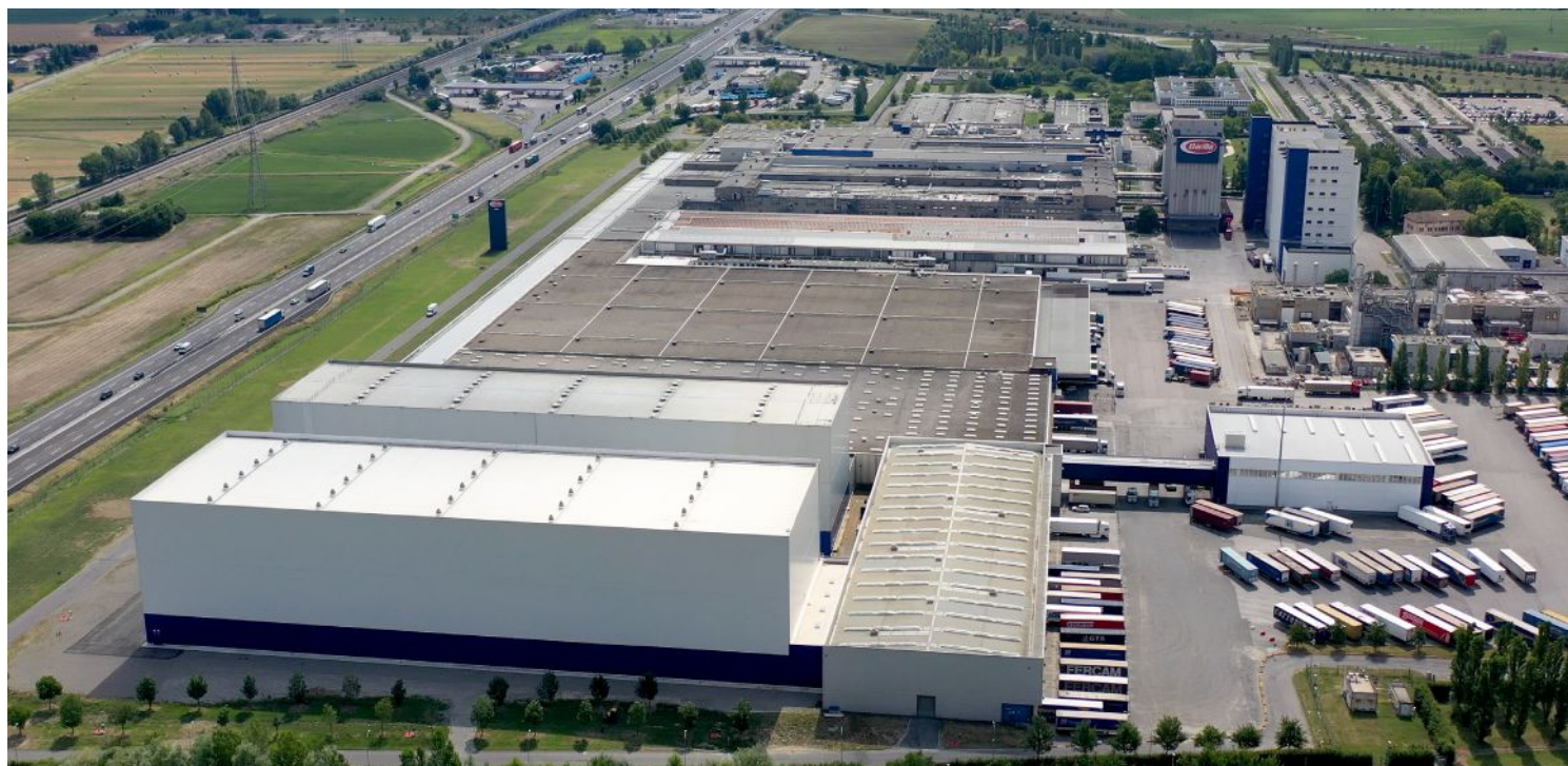
Barilla's flagship pasta production plant in Parma, Italy, is the world's largest pasta products manufacturing site.
