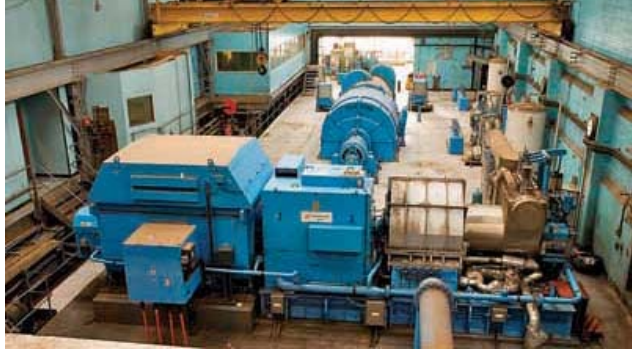
2. The plant's turbine room floor is home to two pass-out turbine generators. The smaller one (just visible in the rear) is rated at 12 MW. The larger one in the foreground is a backpressure unit with a capacity of 35 MW. Courtesy: Slough Heat & Power
