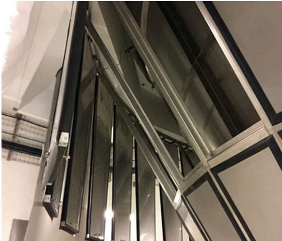
This dryer has removable panels that can be opened and closed easily compared to conventional bolt-on panels. Photo courtesy Dedert Corporation.
