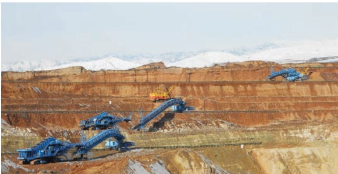
In-pit crushing plant, overburden 5250 t/h, Uzbekistan
