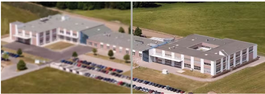
Figure 1: An aerial image of a building is shown with (right) and without (left) image stabilization and resolution enhancement. (Courtesy of PI)
