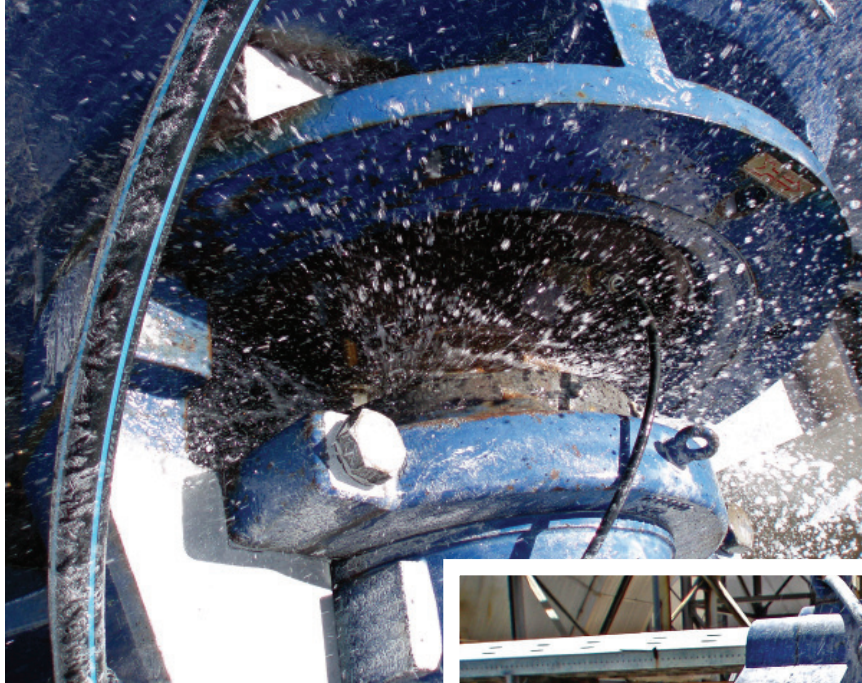
Examples of pump packing seal exhibiting excessive leakage to the environment
