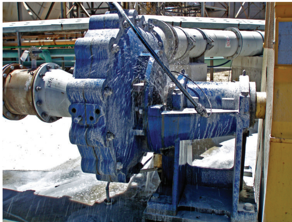
Examples of pump packing seal exhibiting excessive leakage to the environment
