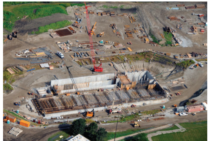
Aerial view of high-rate treatment facility under construction 2
