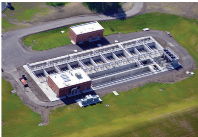
Aerial view of high-rate treatment facility
