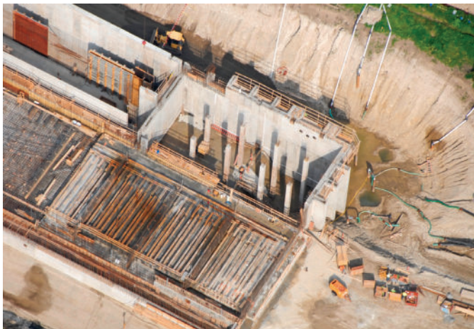
Aerial view of high-rate treatment facility under construction
