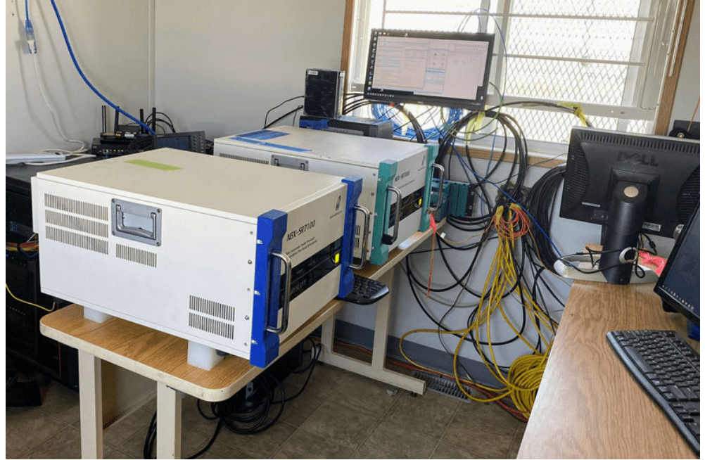
Fiber optic interrogator units that are connected to fibers that run down the wellbore for thousands of feet. Photo courtesy of Neubrex Ltd.
