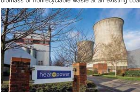
1. Slough Heat & Power's Renewable Energy Center. Courtesy: Slough Heat & Power
