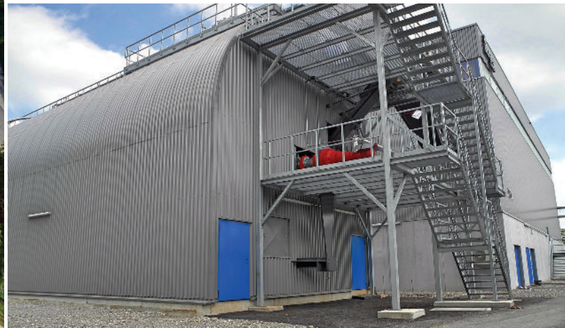
On site, sludge from wastewater digesters supply thermal energy to run the facility.
