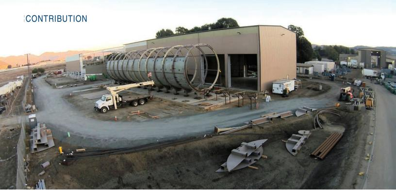
The San Luis Obispo County digester construction is underway. The continuously fed, horizontal PF1800 plug-flow digester has a nominal capacity of 64,000 cubic feet, at a filling level of approximately 85 percent. It is a patented steel structure with inner dimensions of 130 feet long by 28 feet in diameter. PHOTO: HITACHIZOSEN INOVA U.S.A.
