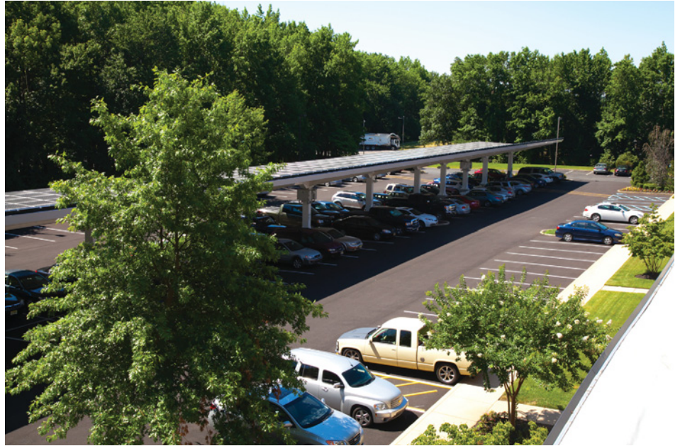
Parking pavilions shade employee cars, and power two electric-vehicle charging stations.
