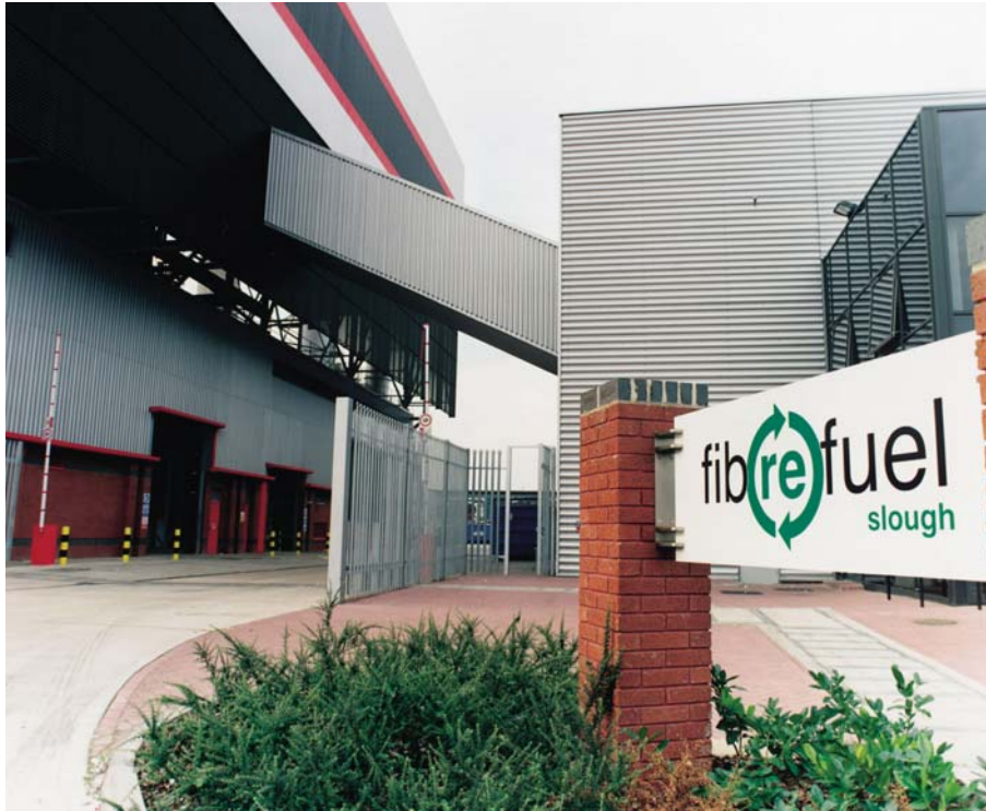
Fibre Fuel plant in the U.K.
