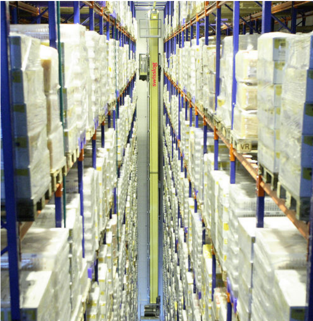
Stacker crane in deep-freeze warehouse
