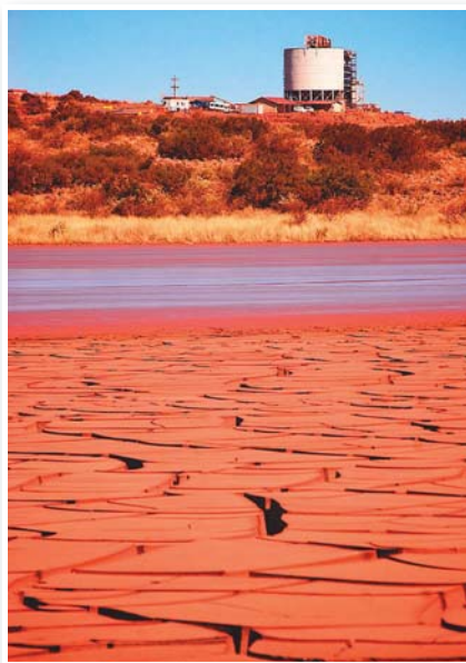
Khumani tailings pond with secondary paste thickener.
