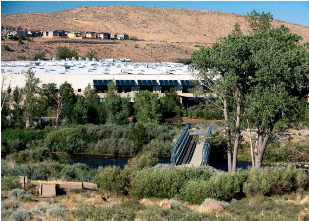
■ The expanded Patagonia distribution center has been designed to reduce its demand on energy and recycle/reuse building materials to create a green facility. Photo courtesy Patagonia, Inc.
