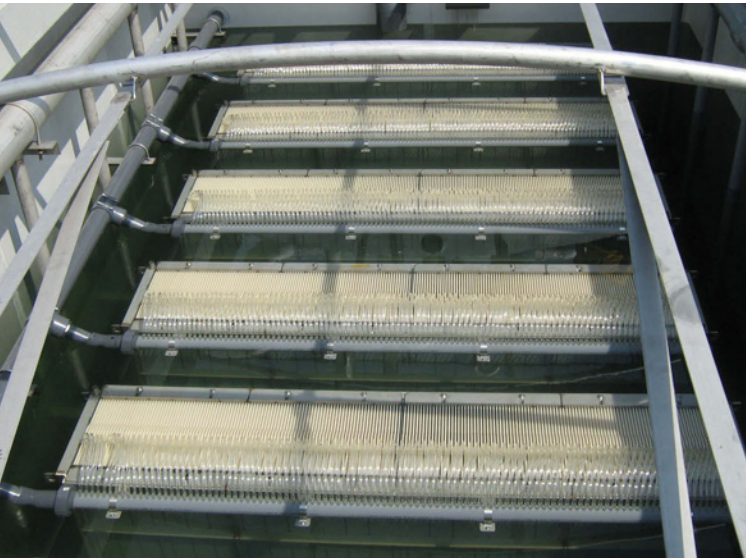
A membrane reactor tank opened for inspection.
