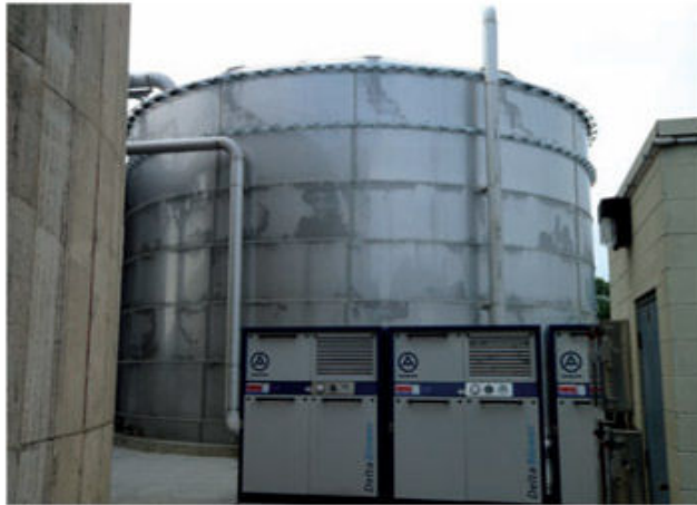
Figure 2: A Control System Integrates the Functions of the MBBRs with Upstream and Downstream Plant Processes.
