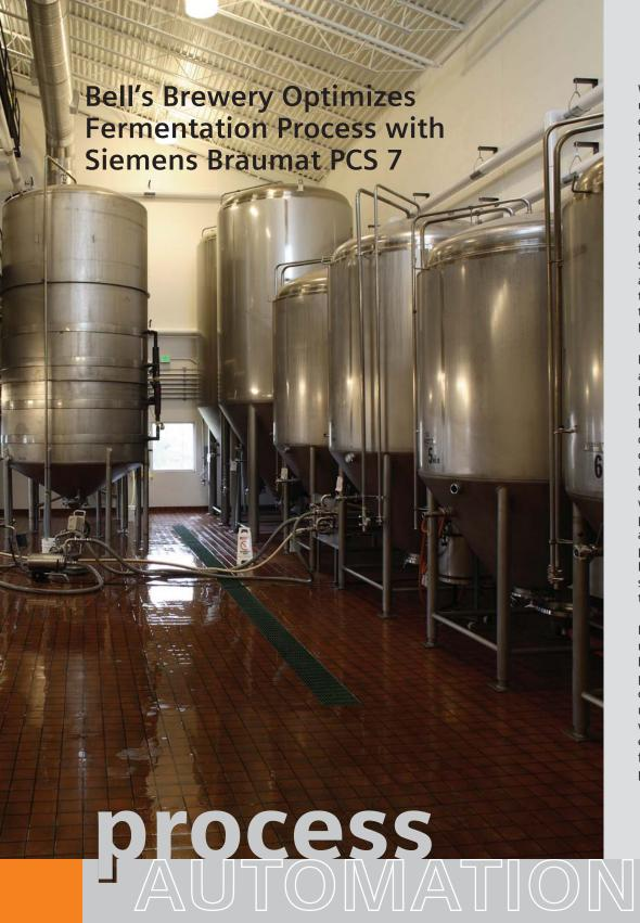
When Bell's Brewery decided to upgrade the temperature control system on its 45 fermentation tanks in mid-2006, they were planning on simply expanding their existing system of dedicated single-loop controllers for each of its tank control points. Instead, Bell's opted to take a quantum leap forward by implementing a state-of-the-art process automation system for temperature control of its tanks – the Siemens Braumat PCS 7 Compact.
