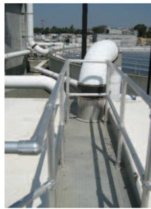
extreme puncture and tear resistance, low thermal expansion and contraction properties, a wide range of chemical resistance, high flexibility, and dimensional stability under high loads and temperature fluctuations, making it ideal for wastewater cover applications.
