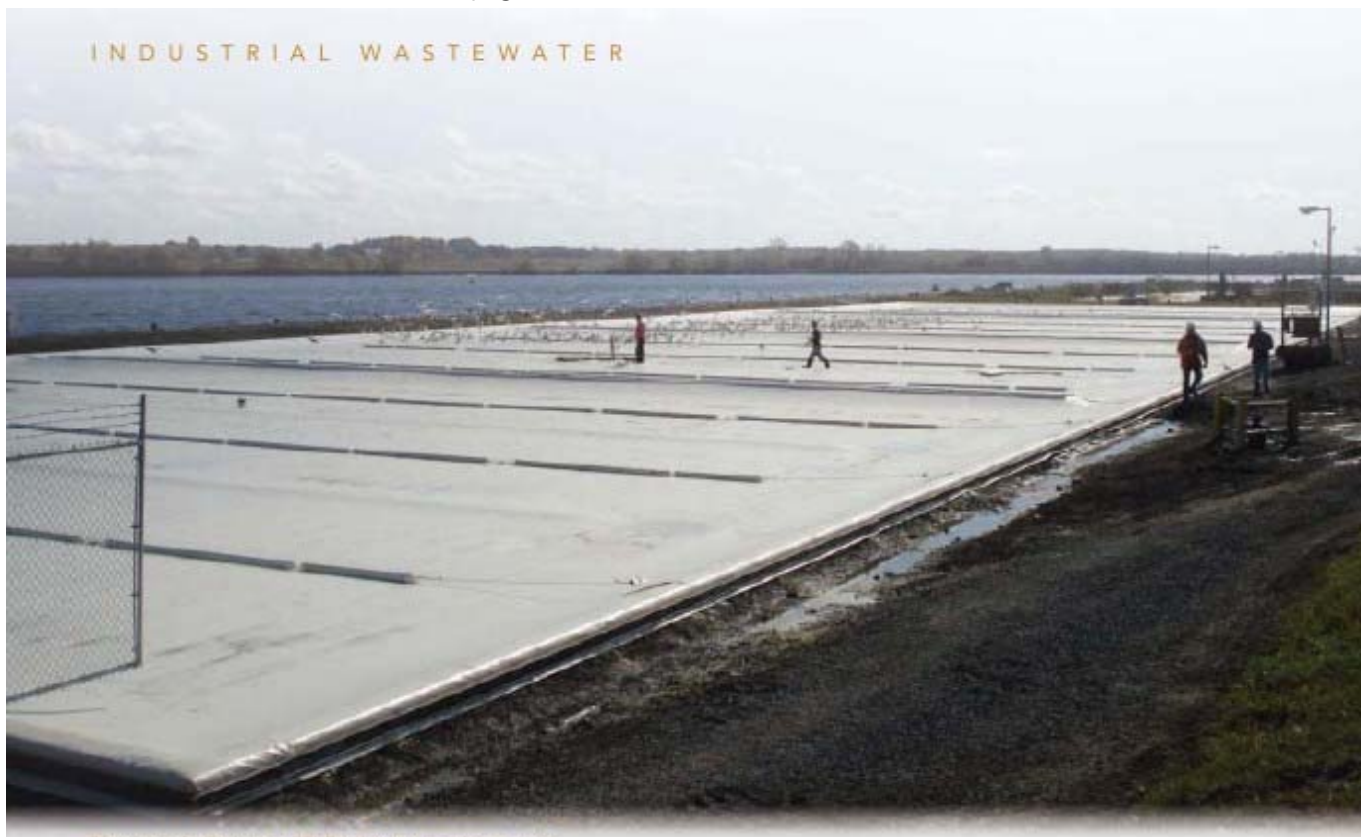
The Casco facility's new GTI floating geomembrane cover
